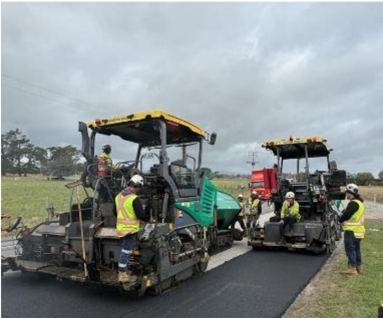
Road rebuild works on SH2 Clareville, May 2026
