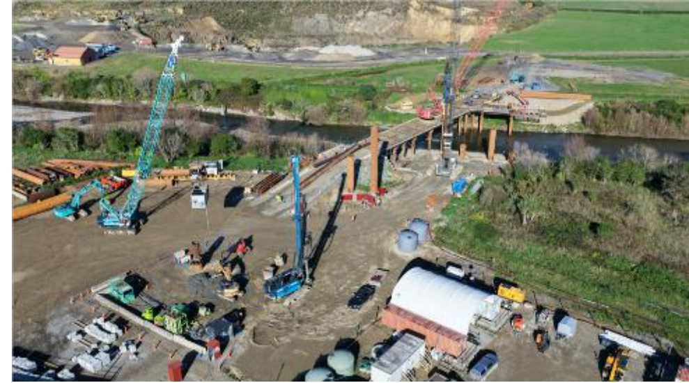
Ōhau River Bridge temporary staging
