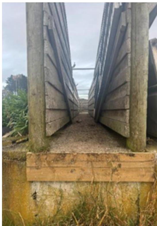
Figure 4. A cattle ramp with a timber buffer
